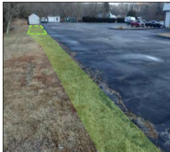
Figure 4.5. Parking lot at Oswegatchie Fire Department looking southeast. Area in foreground indicates the location of a proposed swale to convey stormwater to a proposed bioretention basin (dashes).
