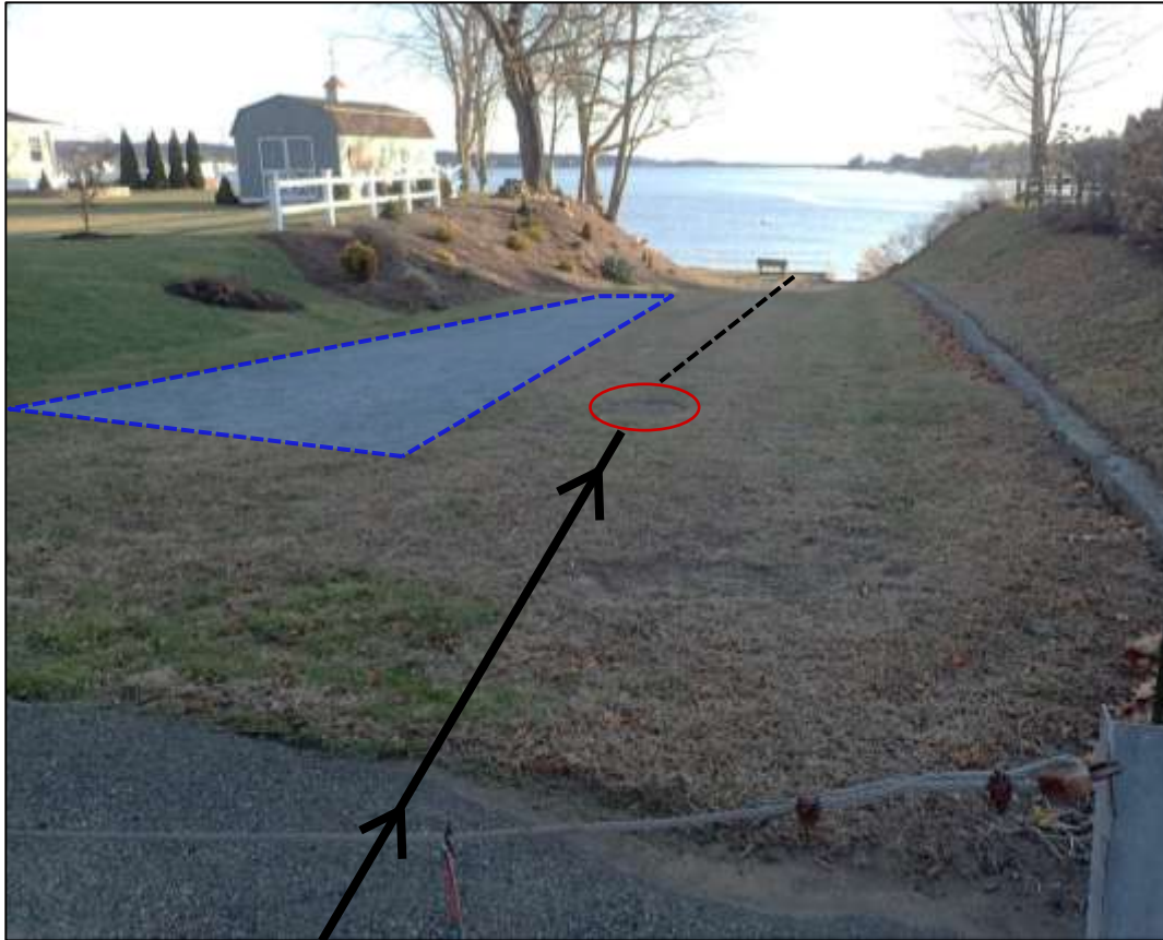
Figure 4.46. Beach access from Park Drive in Waterford. The dashed polygon represents the approximate area for a subsurface infiltration system. The solid black line is the main drain line, and dashed black line depicts the presumed path of the main drain line to the outfall.
